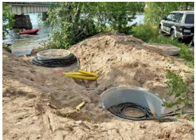
Beachflex™* installation in Finland
